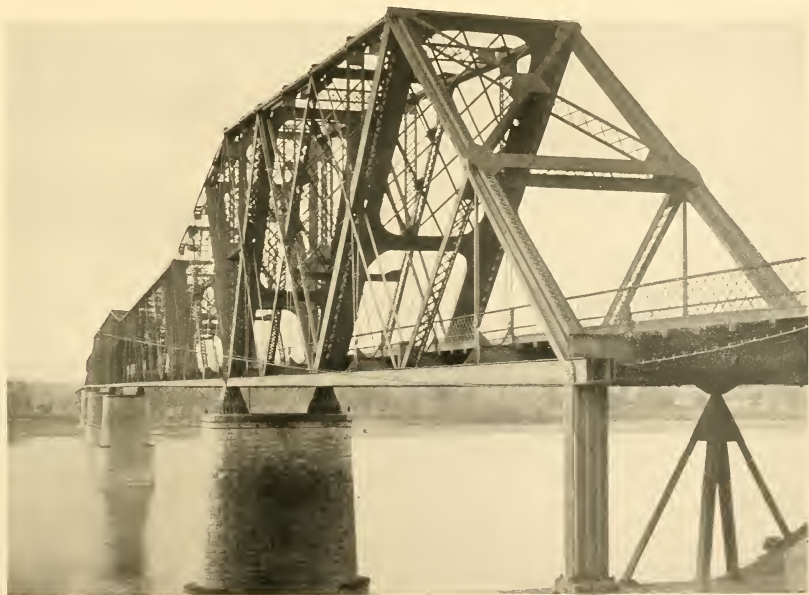
MEMPHIS BRIDGE ACROSS THE MISSISSIPPI
